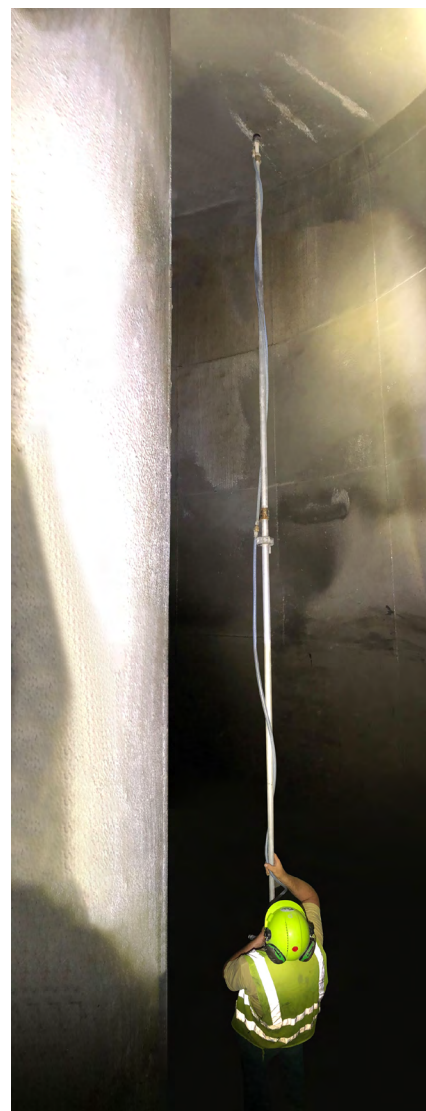
Fig 13 -- A unique pole-mounted sprayer was devised to enable applicators to reach up to 20 ft (6 m) up to apply Xypex Concentrate and Xypex Modified to the saturated surface dry (SDD) concrete of both the large drop shaft and smaller maintenance shaft.
