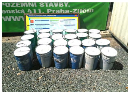
Fig 10 -- Xypex Concentrate in 60 lb (27.2 kg) pails await spray application at a staging area near the Ďáblice sewer system shafts. Both Xypex Concentrate and Modified were used in the project to waterproof and protect the cast-in-place concrete.
