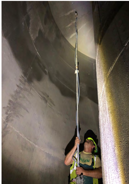
Fig 12 -- Here, a worker sprays Xypex Concentrate to the interior surface of the large drop shaft in the new sewer system serving District 8 in Prague.
