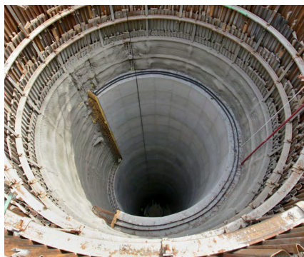
Fig 6 -- The large shaft in the system is 20 ft (6 m) O.D. x 17.2 ft (5.2 m) I.D. x 118 feet (36 m) tall. Shown here under construction, the drop shaft will eventually have a spiral staircase and sewage chute that will allow wastewater to flow in a controlled way to the new transfer tunnel.
