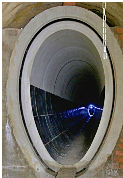
Fig 11 -- Egg-shaped sewer lines are commonly used throughout the city of Prague, the capital of the Czech Republic. A new 820 ft (250 m) long wastewater transfer tunnel was built as part of the new sewerage project for the enclave of Ďáblice.
